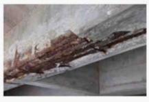
The detection of the hot spots where active corrosion begins - in volves the measuring of the localized nega tive values of the halfcell potential (i.e. corrosion potential). When using a rod electrode the user has to define a grid fine enough not to
